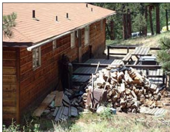
Figure 2. Combustible materials adjacent to a building create a hazard (Anchor Point Group, Boulder, CO).
